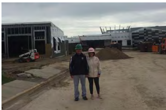
Goldmann and Oglala Lakota Superintendent Anthony Fairbanks touring new construction at Wolf Creek Elementary School, which will be the largest elementary school in the state when completed
